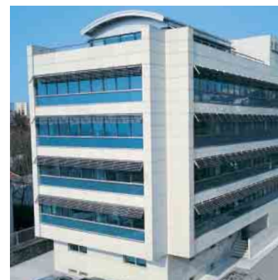
FW 50+ DK, Enka Building, Istanbul, Türkei FW 50+ DK, Enka Building, Istanbul, Turkey
